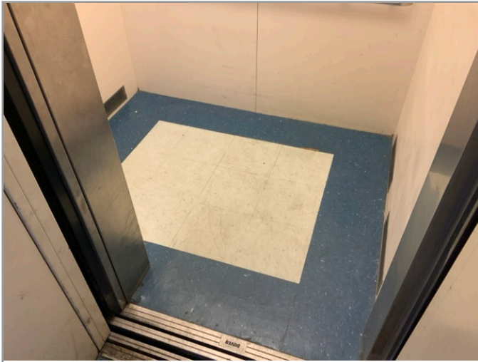
LOBBY LOOKING AT CABS (WITH DOORS OPEN)
