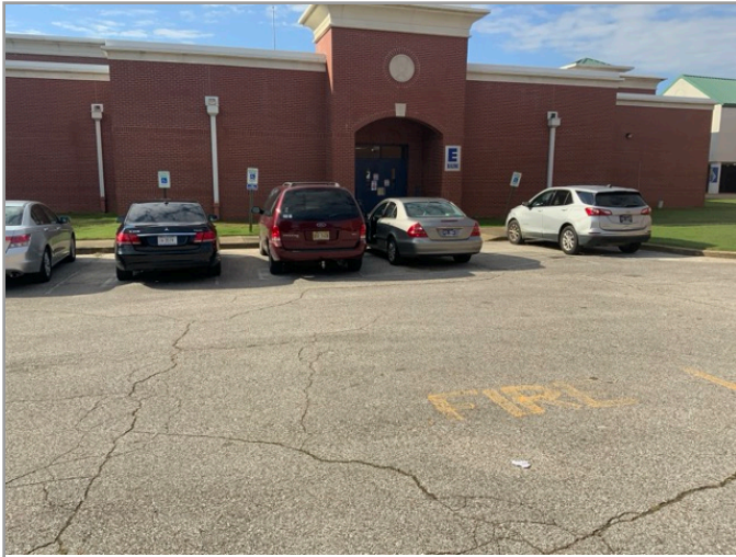
OVERVIEW OF ACCESSIBLE PARKING AREA
