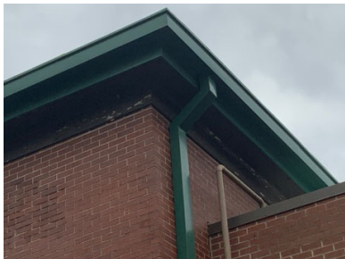
Appears to have dry rot - AssetCALC ID: 8451126
