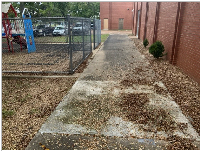
ACCESSIBLE ROUTE TO PLAYGROUND
